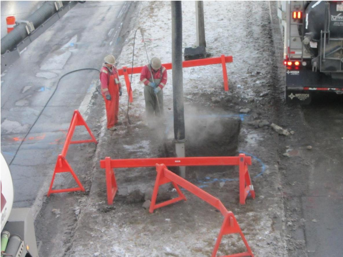
A worker at the site advised that the line break was likely due to corrosion in the pipe, which of course begs the question as to the integrity of the remaining pipe and whether it may soon require additional repairs or even replacement. The City of Calgary has published an information brochure (inserted below) that lists the primary causes of water main ruptures. These primary causes include:
